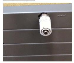
All radiators are provided heated water from the boiler based on the integrated building heating, ventilating and air conditioning building management system per set points as noted above. Each radiator on the perimeter has its own integral thermostat that the occupant can adjust.
